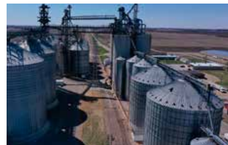
Grain assets in Beltrami, Minn., are some of the assets that are now part of CHS West Central.
