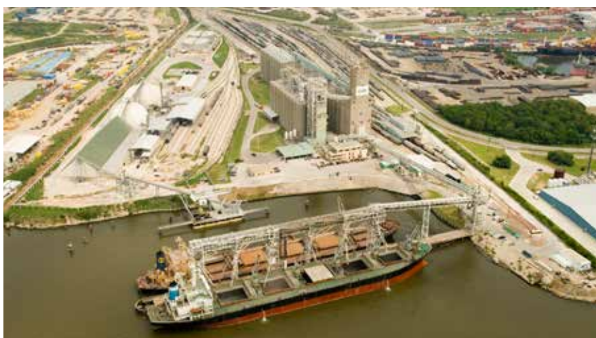
CHS and Cargill plan to expand their TEMCO joint venture by adding the Cargill-owned export grain terminal in Houston, Texas. (Photo courtesy of Cargill.)
