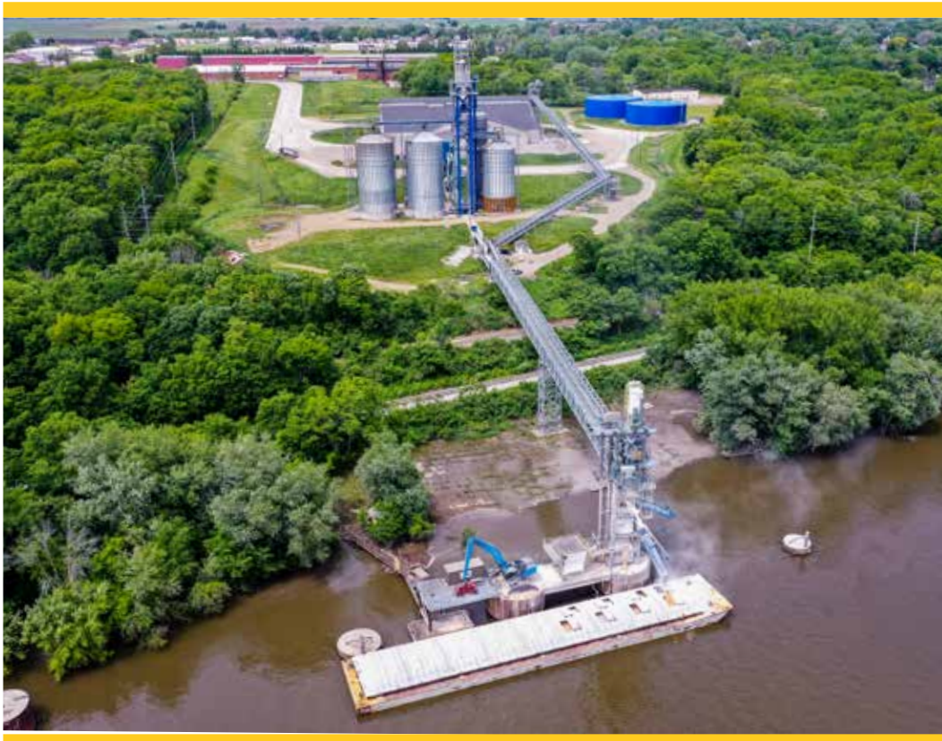
The CHS terminal in Peru, Ill., sends corn down the Illinois River to the CHS terminal in Myrtle Grove, La. From there, corn is sent to global markets.
